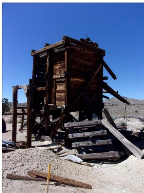
Richardson Mine shaft
